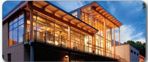
The Albert M. Higley Co. employs 84 full time salaried employees in their Cleveland and Columbus offices. One recent project was constructing a new training facility for the Cleveland Cavaliers (pictured above).
